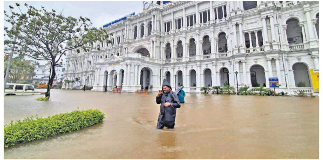
A man wades through a waterlogged road outside Ripon Building during heavy rain owing to Cyclone Michaung, in Chennai. — Photo: PTI
