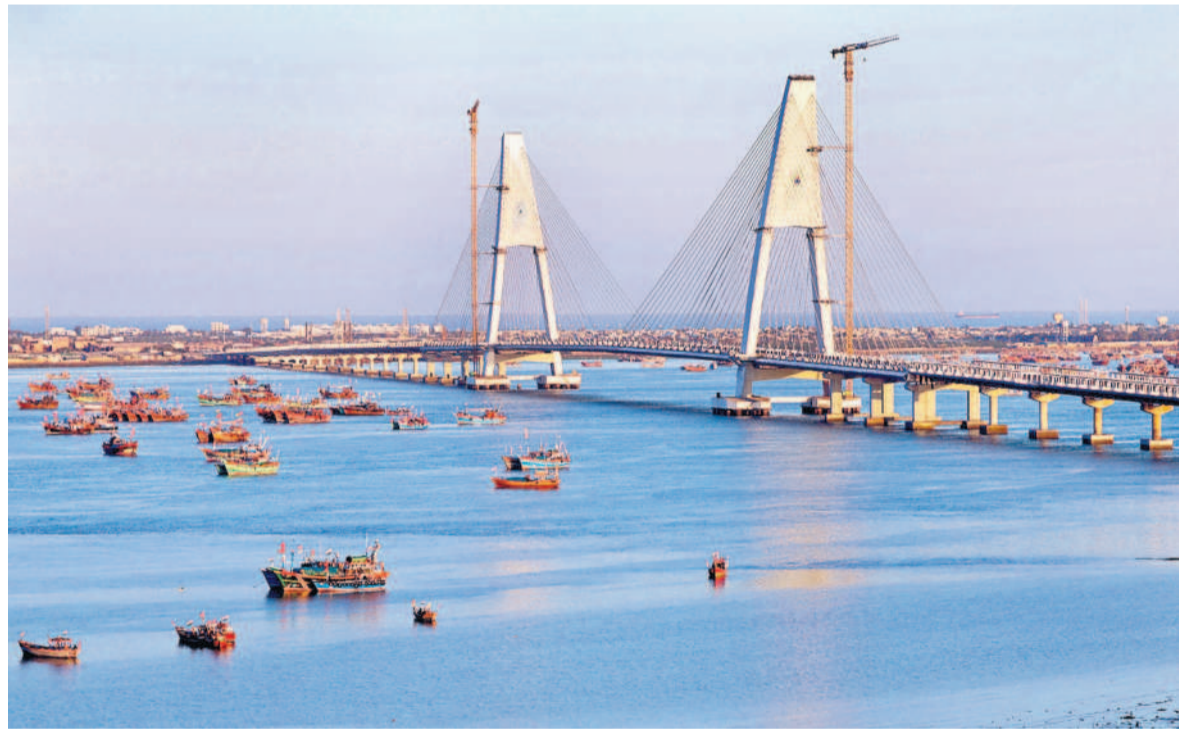
NEW LANDMARK: Sudarshan Setu, India's longest cable-stayed bridge, was inaugurated by Prime Minister Narendra Modi on Sunday in Gujarat. The bridge, connecting Okha mainland and Beyt Dwarka island, boasts of a unique design, featuring a footpath adorned with verses from the Srimad Bhagavad Gita and images of Lord Krishna. — Photo:PTI
