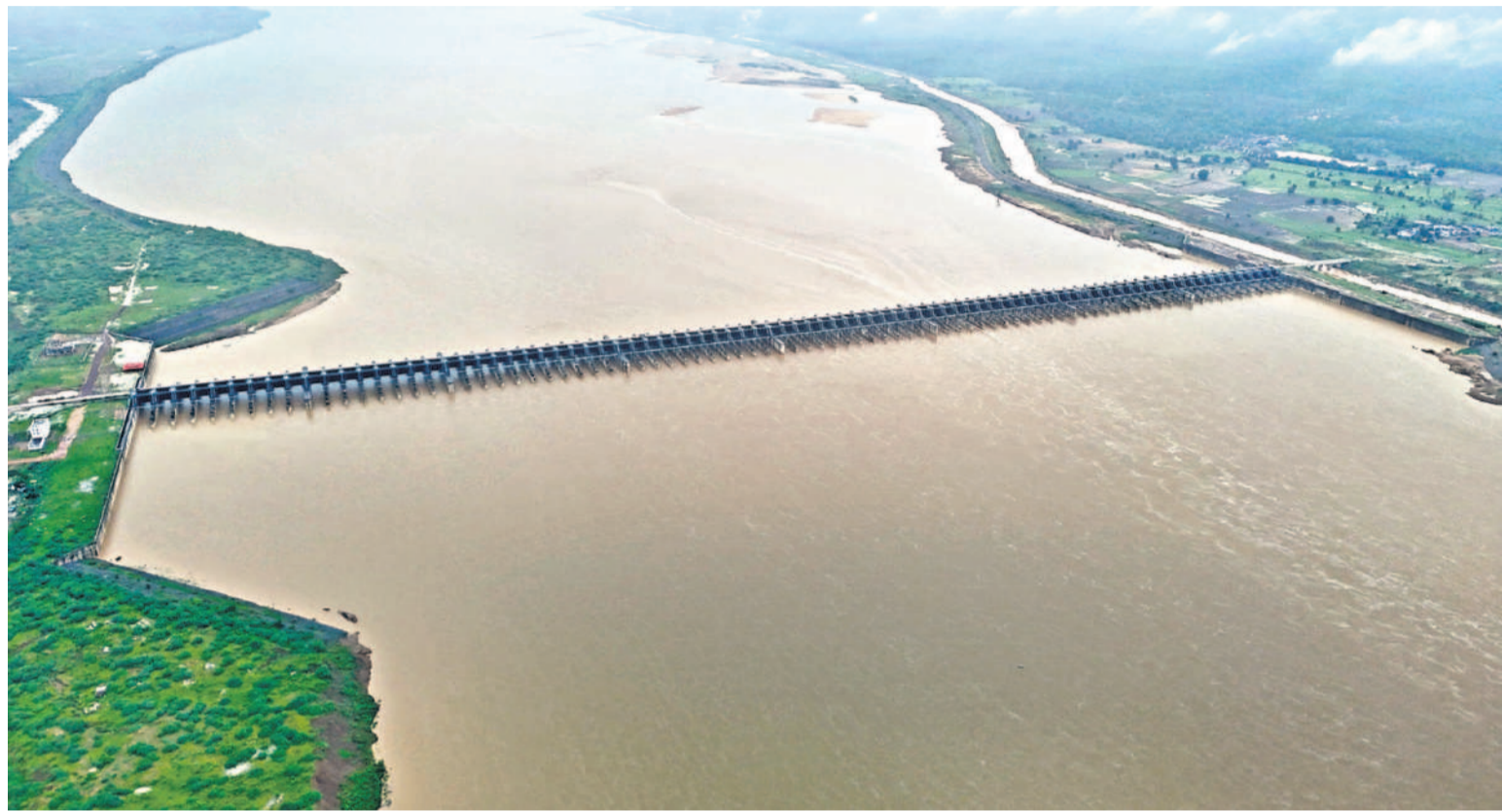
The barrage, with all its floodgates opened, is able to discharge over 3.7 lakh cusecs of water even at the impacted piers.
