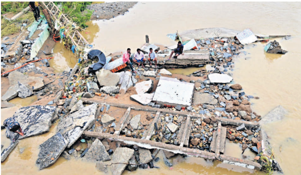
People sit on a structure which collapsed due to heavy rains that lashed the State, in Khammam on Monday.
