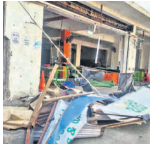
HYDERABAD | PAGE 03 HYDRRAA demolishes commercial units in city
