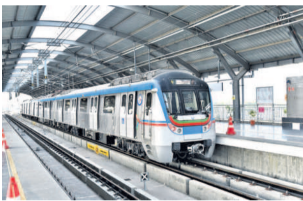
The two corridors were initially proposed by the previous BRS government from Paradise to Kandlakoya and JBS to Thumkunta as two levels or a double-decker flyover.
