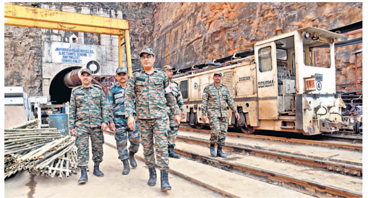
Army personnel near the SLBC project site where a portion of the tunnel collapsed, in Nagarkurnool district on Monday. — Photo:PTI
